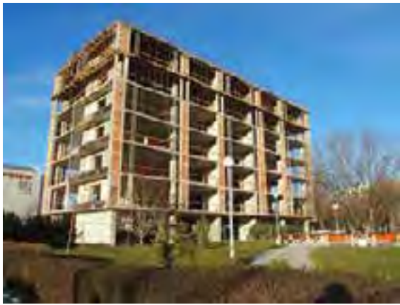
Fig. 6. The example building as an example for avoiding torsionally flexible system
