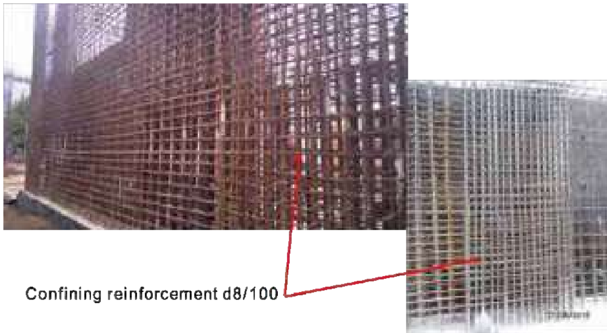
Fig. 24. Reinforcement detailing requirements for DCH
