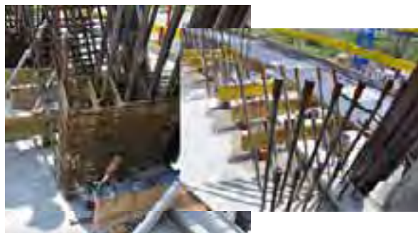
Fig. 36. Application of splicing devices for longitudinal bars in a RC building designed and detailed according to Eurocodes
