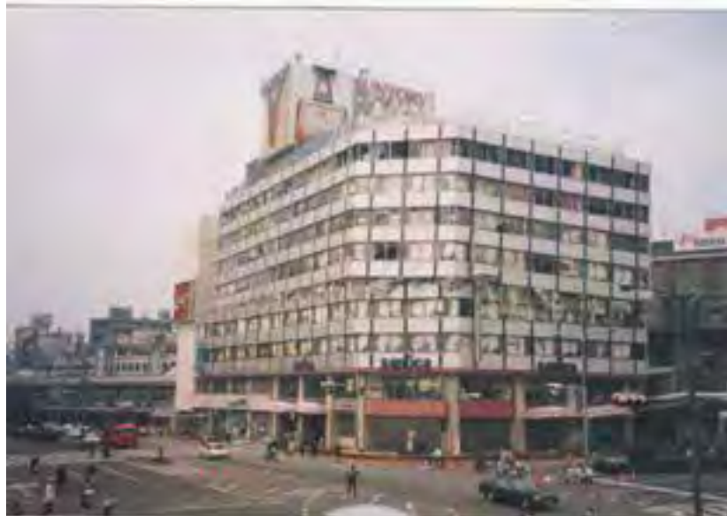
Fig. 5. Heavy damaged office building with torsionally flexible system during the earthquake in Kobe 1995
